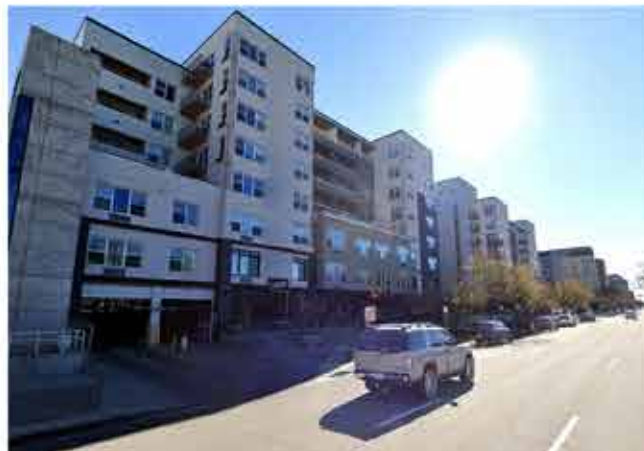
⑥ ON GRANT STREET LOOKING EAST
